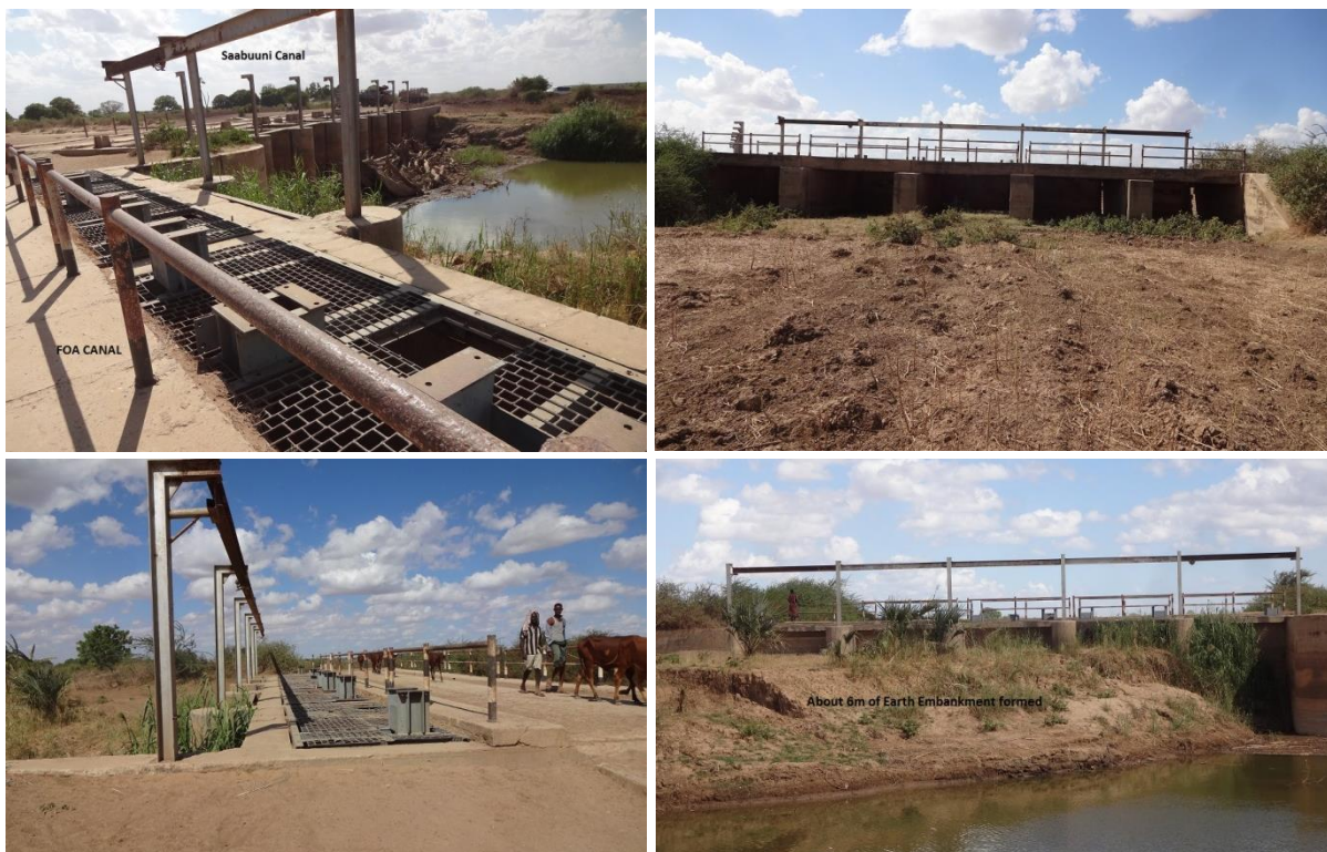
Figure 3-6 Upstream and downstream of supply (FAO) canal and head regulator
