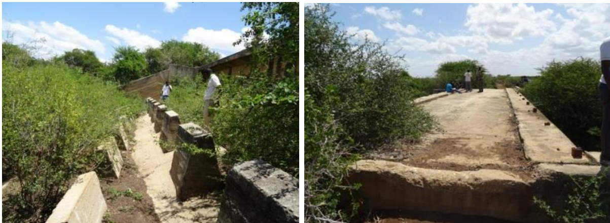
Figure 3-7 Photo shows supply (FAO) canal outfall structure (Source: WOCCA)
