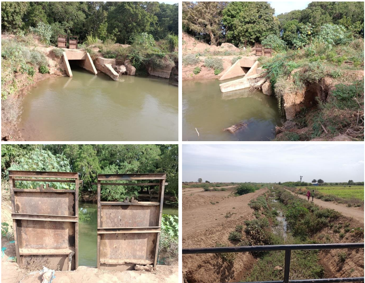
Figure 3-14 Intake structure and down reaches of Labaa Primary Irrigation Canal
