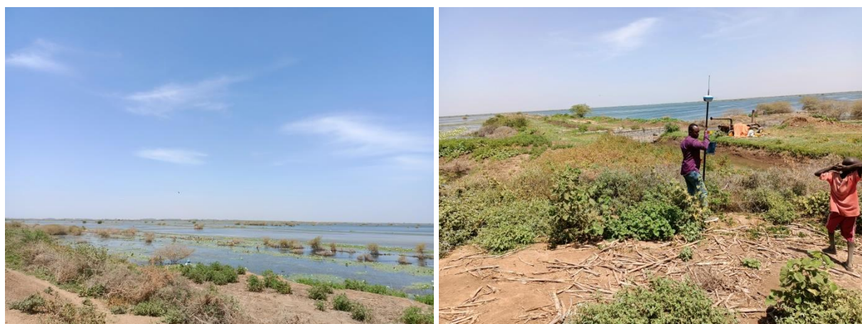
Figure 3-8 Photo shows Jowhar off-stream storage reservoir and embankment
