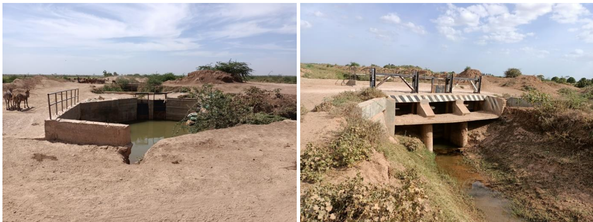
Figure 3-16 21st October primary canal intake structures
