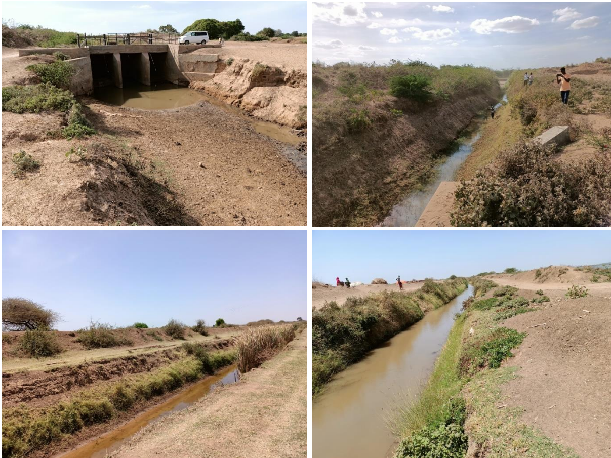
Figure 3-17 Intake, upper reaches and tail escape of 21st October Canal into supply canal
