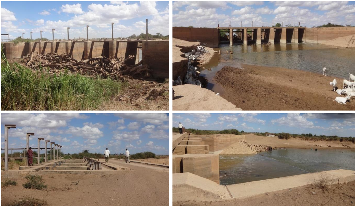
Figure 3-4 Upstream and downstream of Sabuun Barrage
