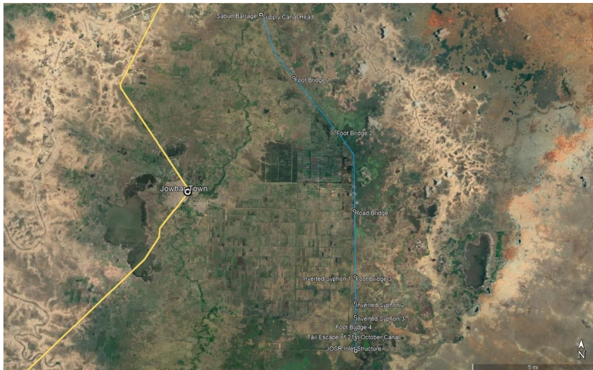
Figure 3-5 Sabuun Barrage, supply (FAO) canal and head regulator
