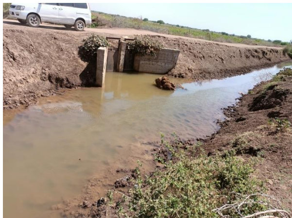
Figure 3-18 Intake structure and down reaches of Kalundi Primary Irrigation Canal
