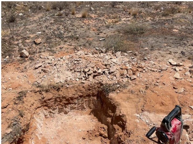
Fig-8: Trial pits excavated with jack hammer
