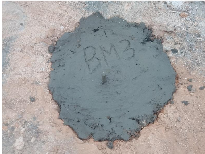
Fig-5: Typical view of the 5 concrete benchmarks casted on 3/5/2024
