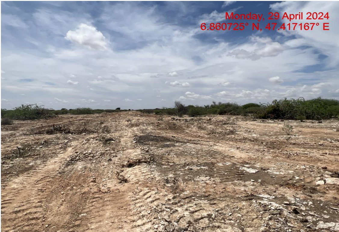
Photo 1. View of the access road under construction at the project site
