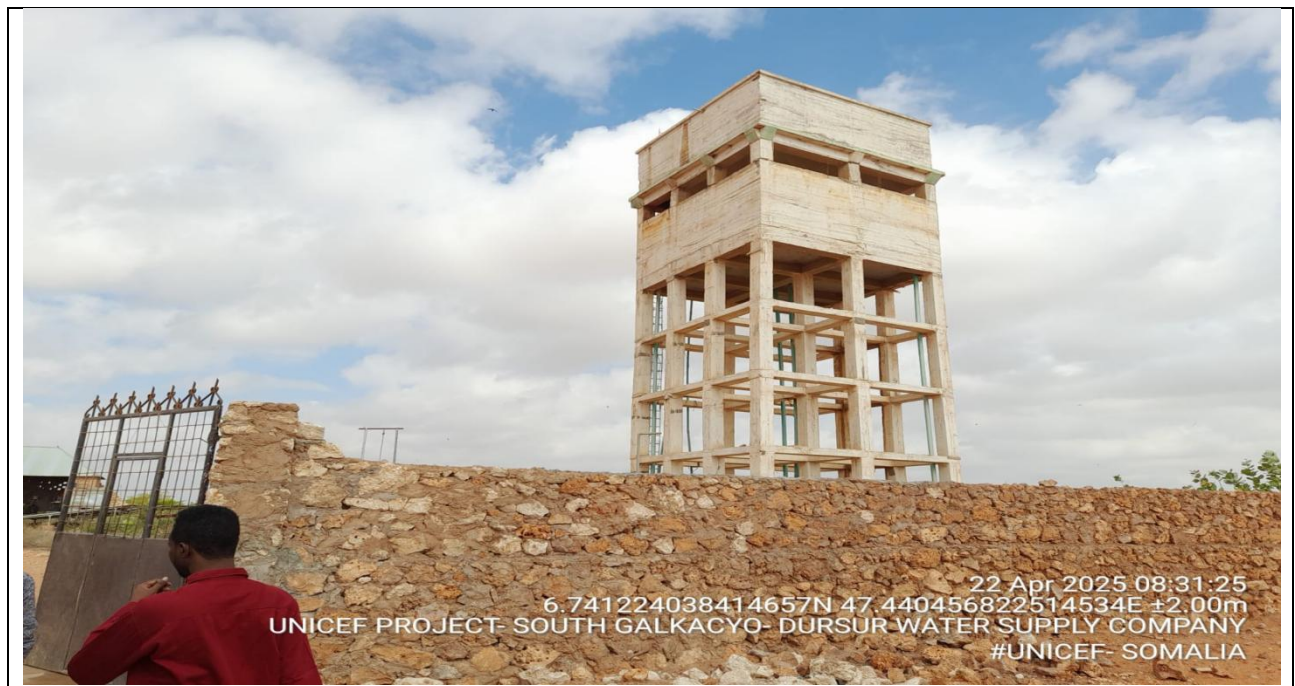
Figure 3-9: Concrete water tank for Borehole for Durdur Water Co. Ltd
