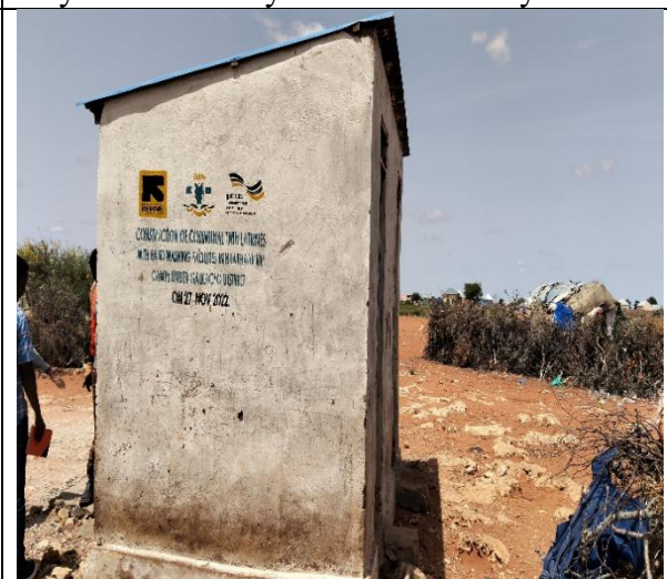
Sanitation facilities in the one of the camps
