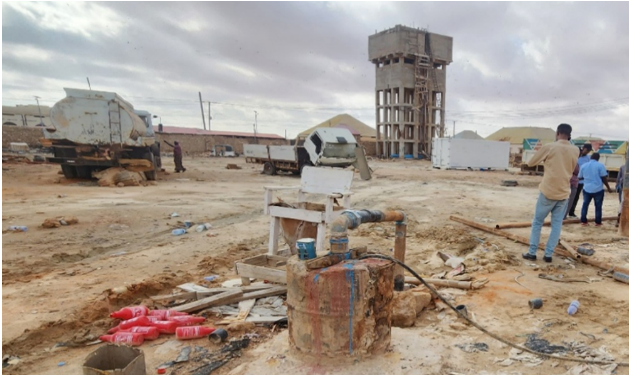
Figure 3-14: Borehole site for Arafat Water Co. and the concrete water tank in the background
