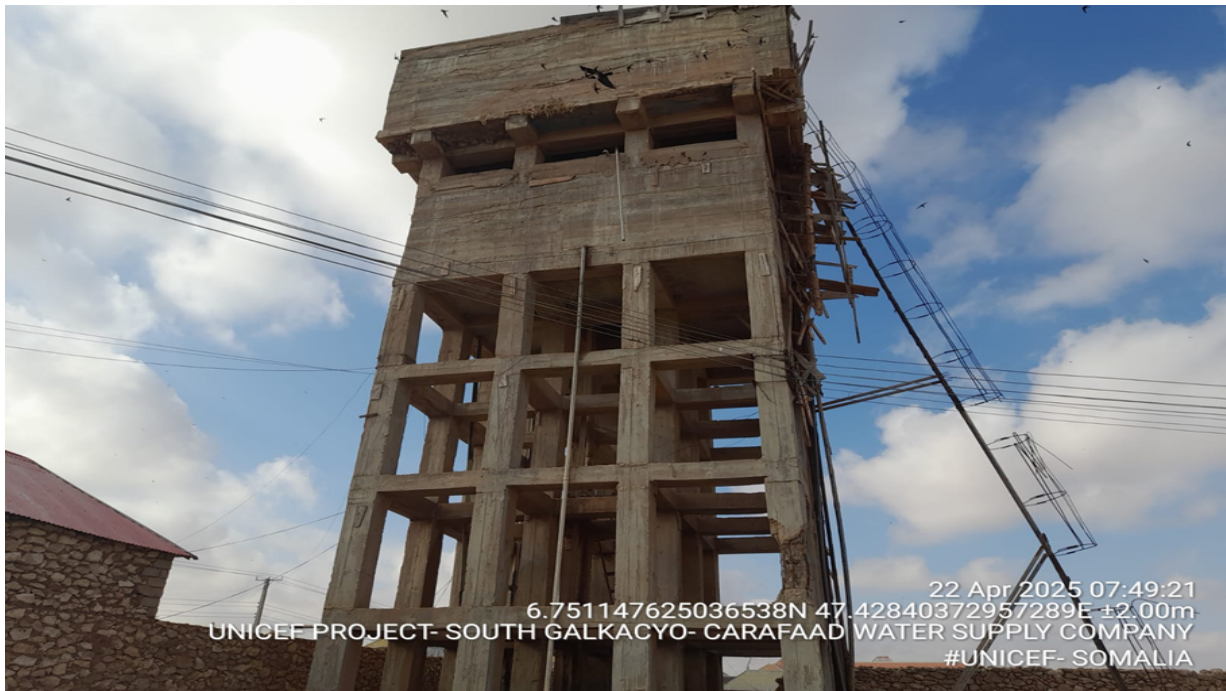
Figure 3-15: The elevated concrete water tank for Arafat Water Co.
