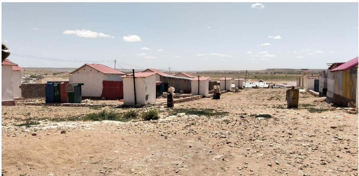
Figure 3.9: Stone build Shared communal pit latrines within Shabeele IDP Camp
