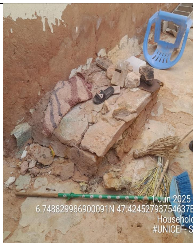
Figure 3.8: Unlined Septic tank in South Galkayo Residential Household.
