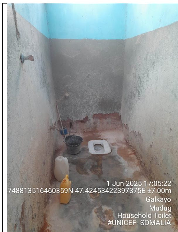
Figure 3.7: Pour flush Toilet in South Galkayo Household.
